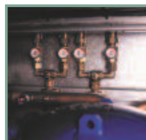
Dual pressure relief valve
