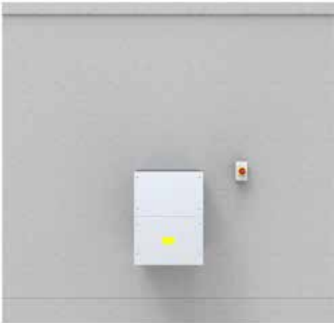
Local Isolator (Typical Placement)
