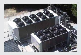
I believe we are the first company in the world to install a TurboChill™ FreeCool chiller. When the data centre is operating in free cooling mode, the PUE has been measured at 1.36 and we expect that to reduce further as we install more equipment.
